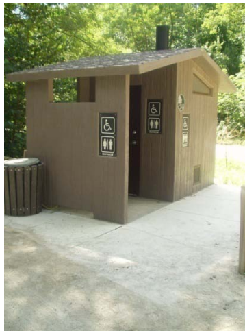
Vault Toilet Facility Clarkston/Kern Roads and the Paint Creek Trail Orion Township 2006
